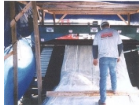
Resin is shown being introduced into the liner.
