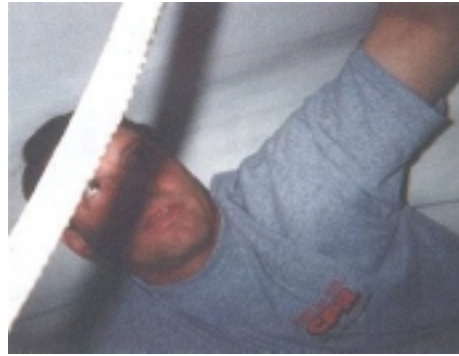
Kerry Coker examines ropes inside the liner to assist with installation.
